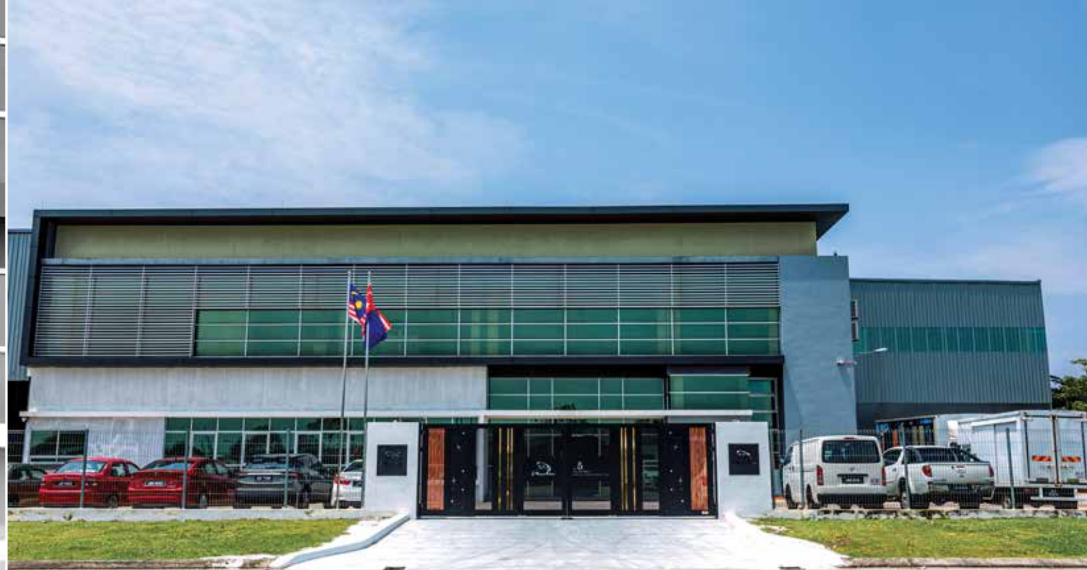
BUILT ON TRUST . EXCELLENCE IS MUST
